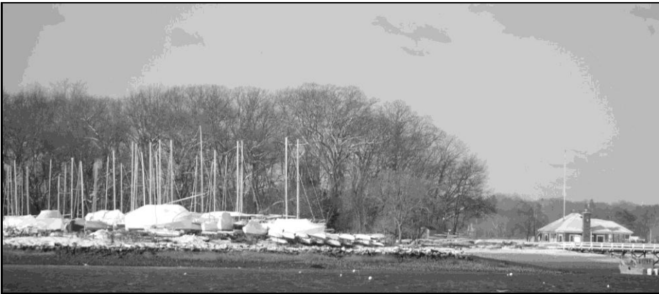
View of the Old Greenwich Yacht Club. A new concrete wash pad is located in the boatyard area.
